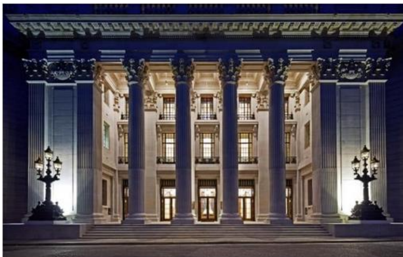
10 Trinity Square in the City which has been turned into a Four Seasons hotel and flats
